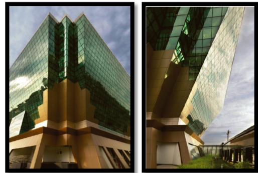
Figure 12 Low-e Glazing Façades (source: Lin Ho. Courtesy of Senandung Budiman Sdn. Bhd)
