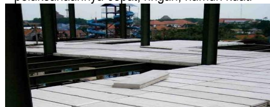
Gambar 8. Panel Plat Lantai AAC ( Autoclaved Aerated Concrete )
