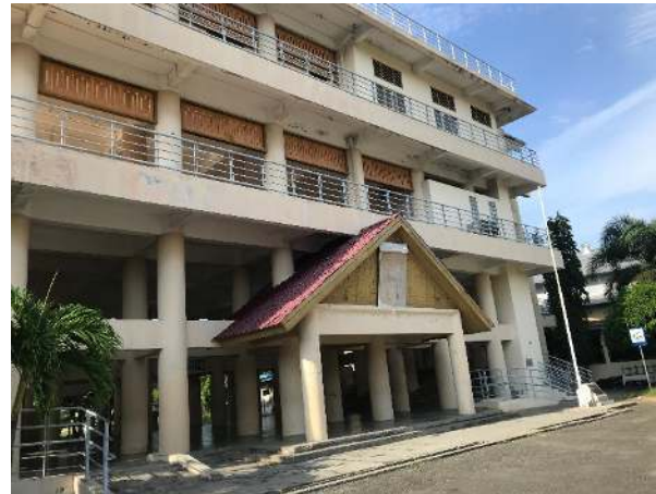
Gambar 2. Escape building Gampong Lambung
